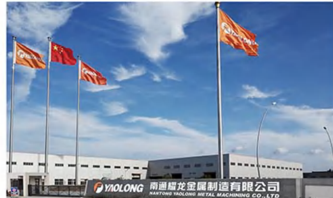
Yaolong Nantong Factory Gate
