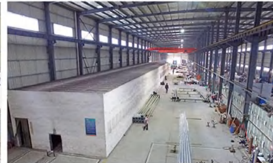
Yaolong Foshan Factory No.2 Inside View
