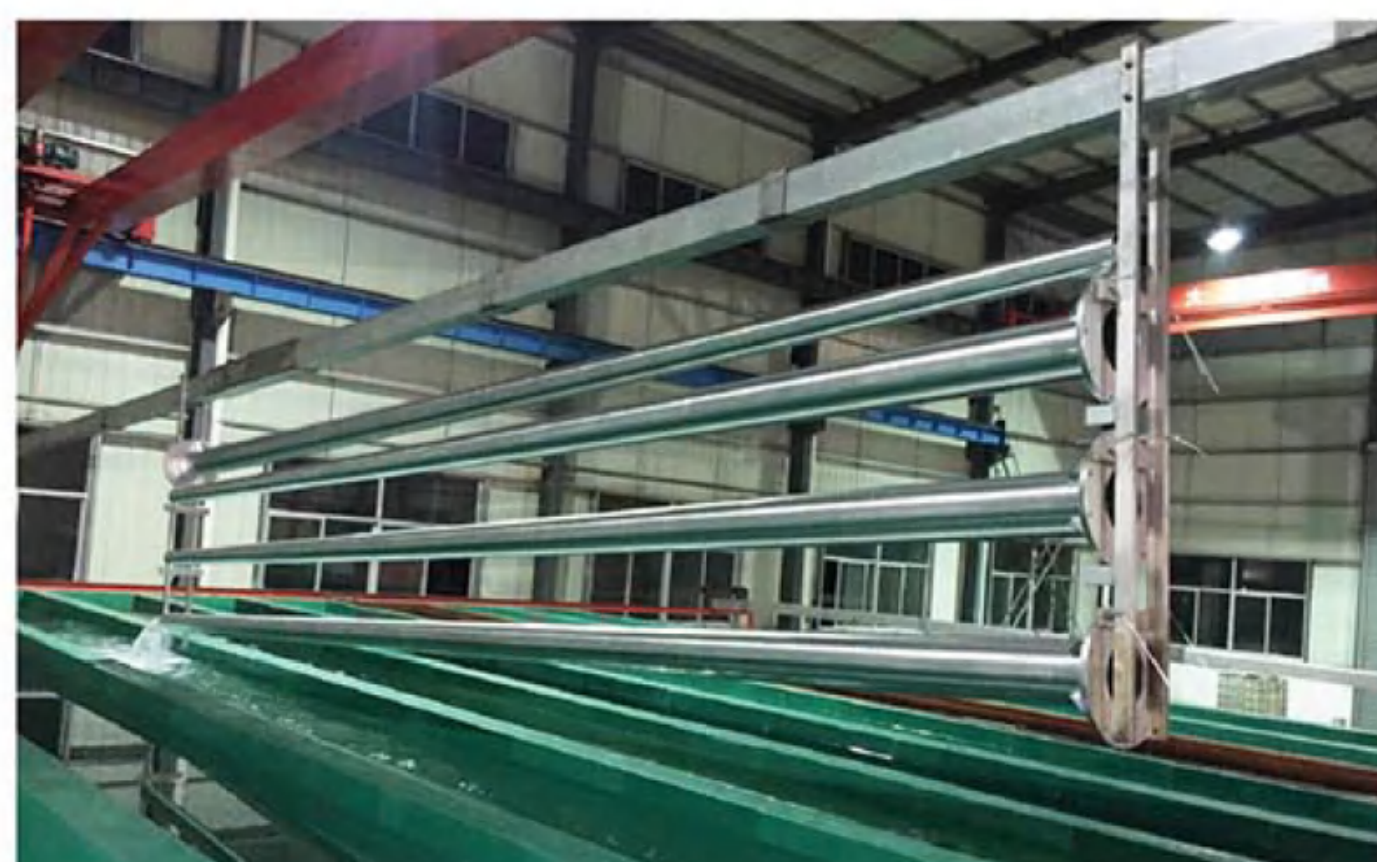
15Meter Long Aluminium Pole Anodizing Pond
